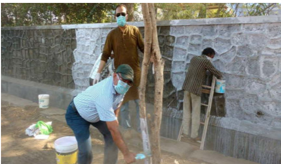
Painting the Walls
